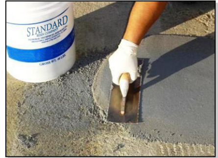
Patching & Resurfacing Concrete
